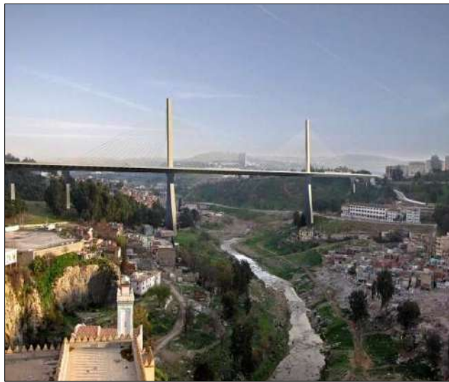
Photo 3. The Trans Rhumel viaduct 119 m its pylons are erected in an unstable area
