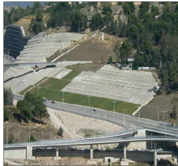
Photo 4. Drainage galleries were made, for the evacuation of groundwater
