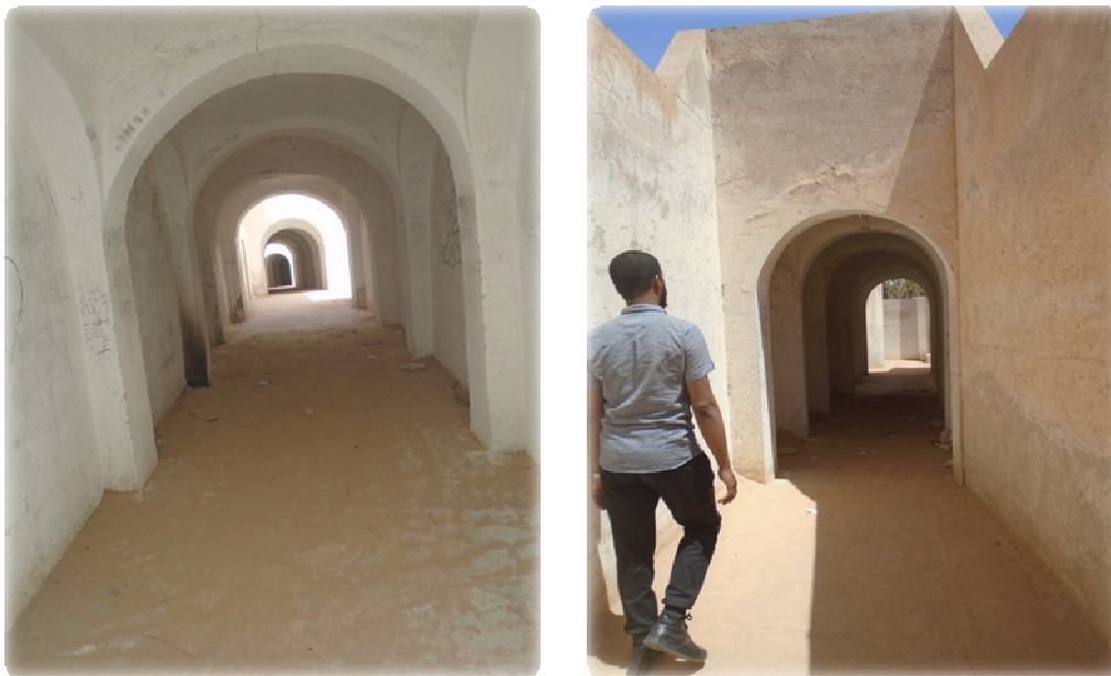
Figure 7: Views of a semi-covered passageway at Tamerna kadima (Oued Righ). The photos show that the streets have sunny and shady areas creating an artificial breeze in summer. Source: Authors, 2019.
