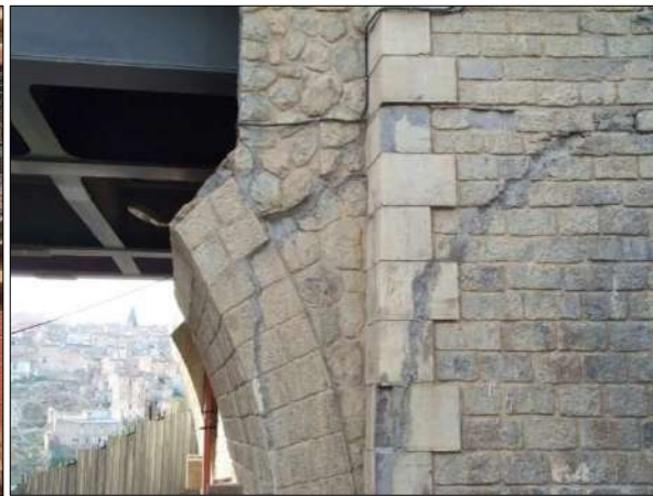
Photo 2 .The Sidi Rached bridge on the right bank of the Rhumel
